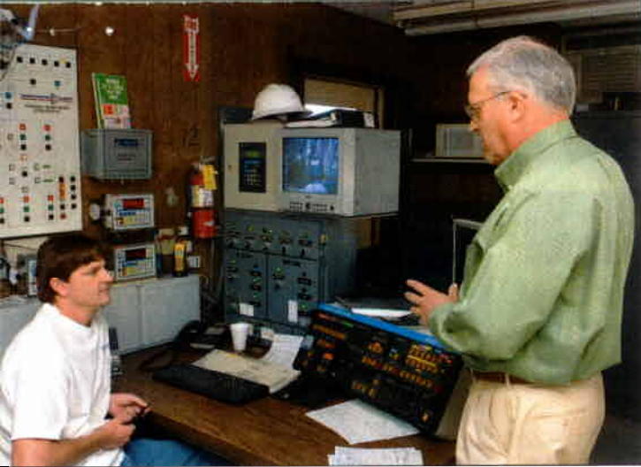
Left: Batchman Richard Bowman (left) talks with Tim Toland, president of National Ready Mixed Concrete Co., at its plant in Van Nuys, Calif.
